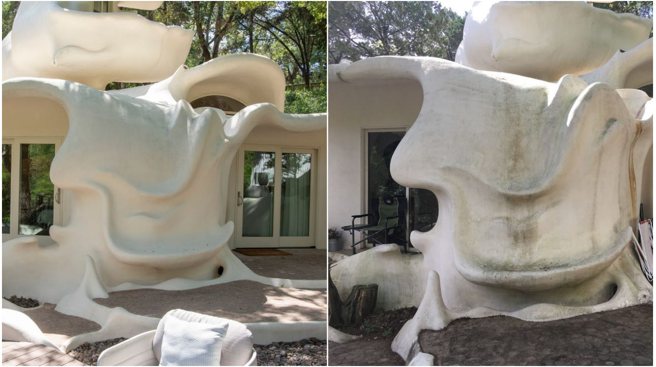
Left to right: The exterior of the Bloomhouse after renovations and before renovations. Courtesy of Dave Claunch via BI
